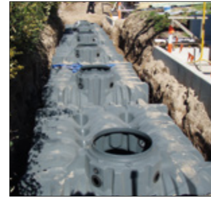
Shopping centre, Geelong (Australia)
