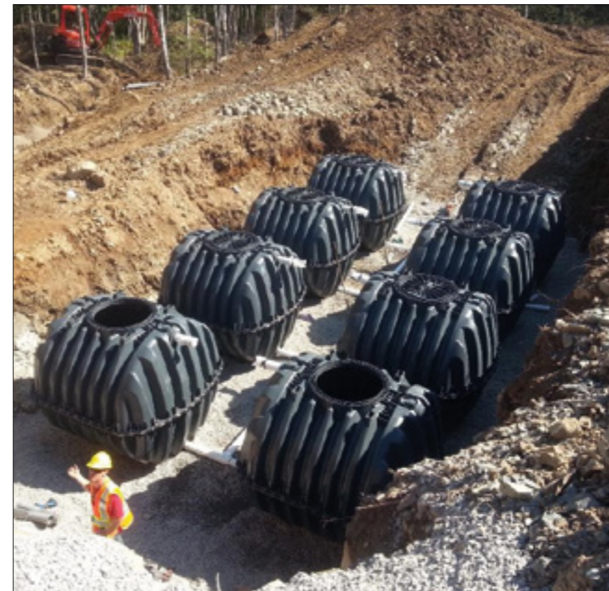
Industrial building, Nova Scotia (Canada)
